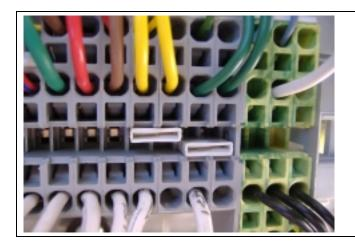
On one occasion the metal insert has pushed up in the plastic housing when the jumper was inserted to the wago block, causing a very poor connection.
